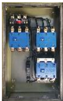
Interior View of ML FASD
