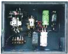
Interior View of MR-G2W
